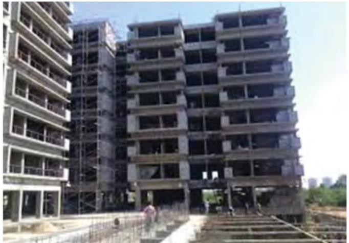
Under construction project in Surat
